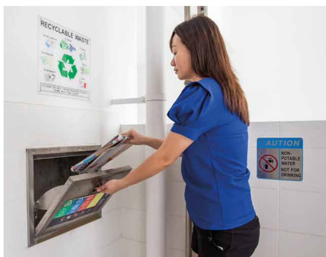
Separate chutes for recyclable waste
