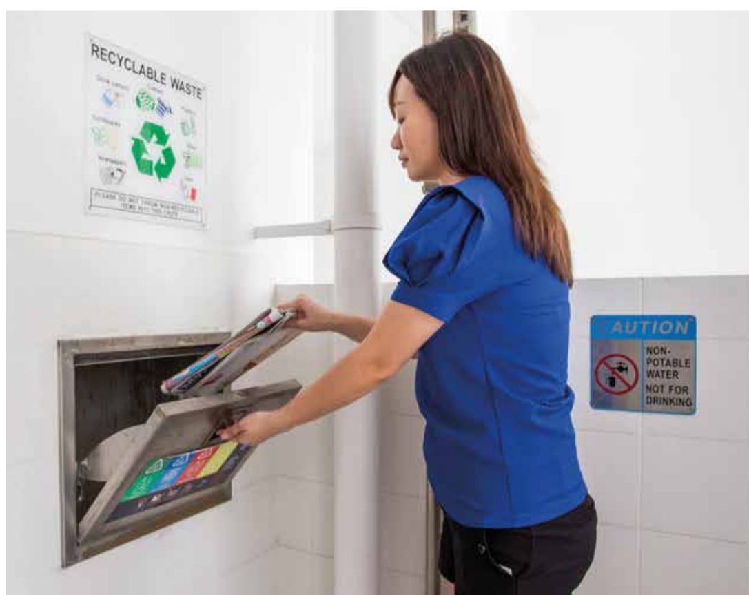
Separate chutes for recyclable waste
