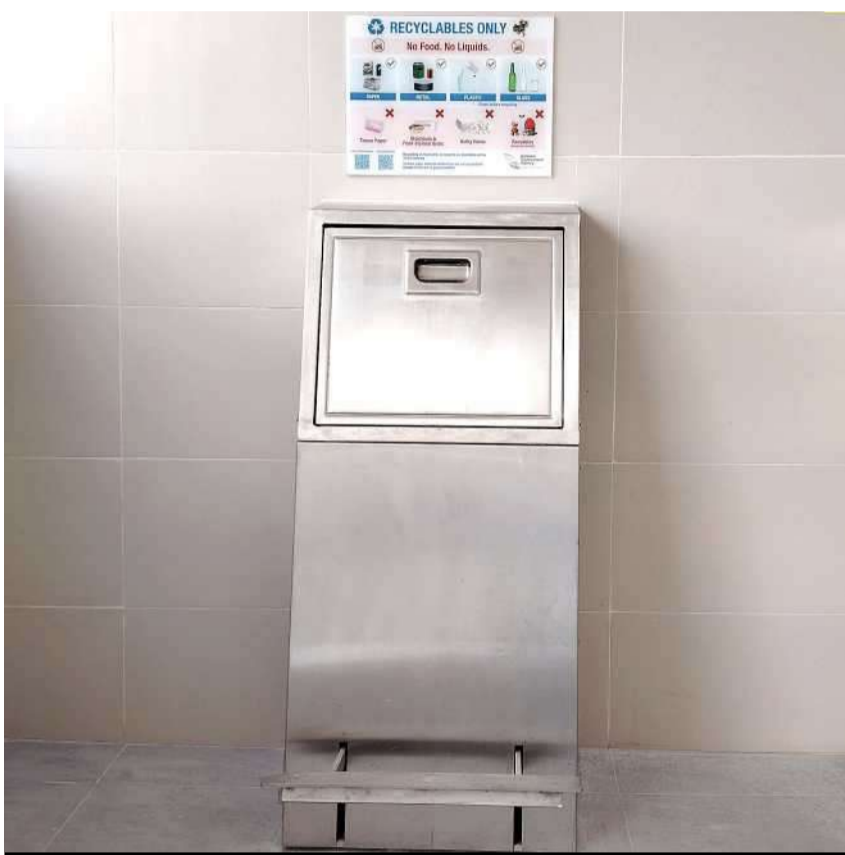
Separate chutes for recyclable waste
