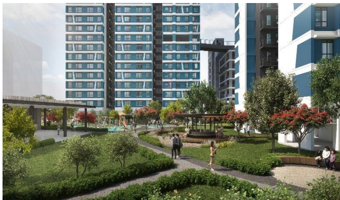
Precinct Green, Precinct Pavilion & Play facilities
