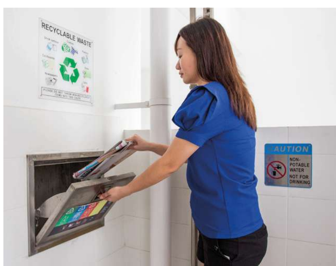
Separate chutes for recyclable waste
