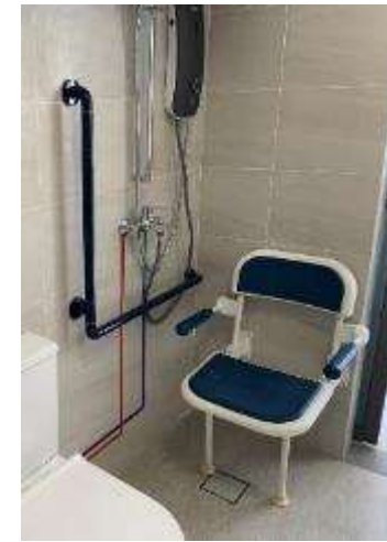
Foldable Show Seat: Installation of shower seat in Bathroom
