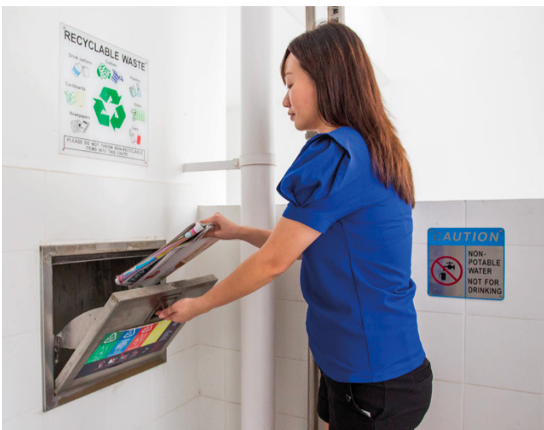
Separate chutes for recyclable waste
